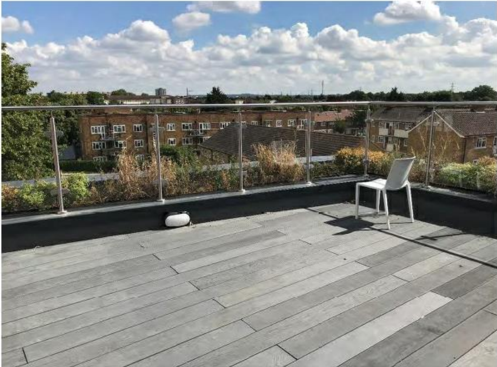
Photo 6: Communal Roof Terrace, fronting onto Chesnut Road
